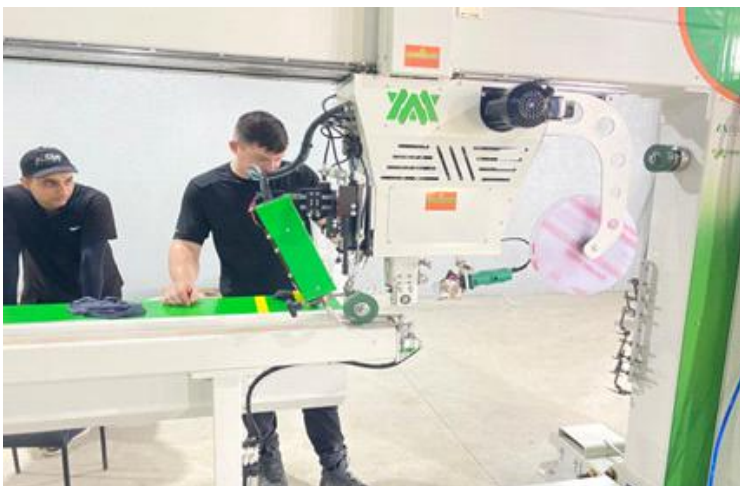
Commissioning of Miller Weldmaster 112 Extreme Machine at M/ S Nithiya Sai Metals LLP, Chittoor
