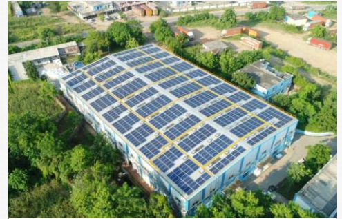
Solar plant installed at Nalagarh
