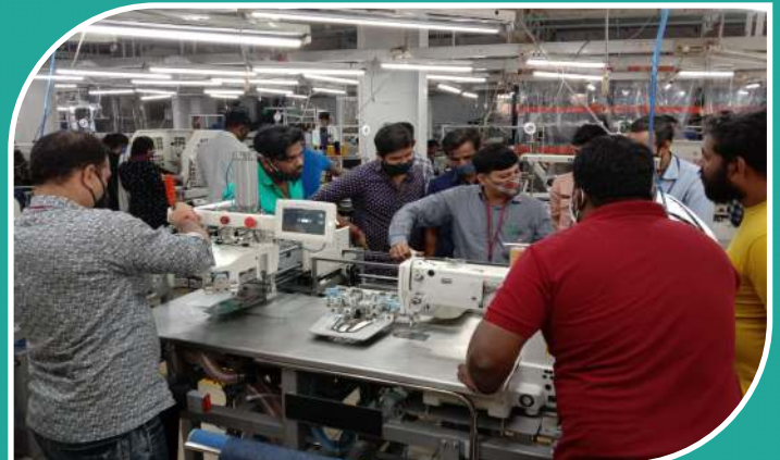
Machine Installation in progress
