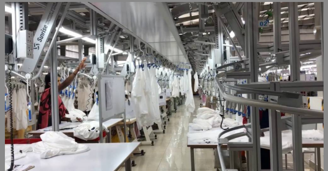
Installation of Sunrise Hanger System
